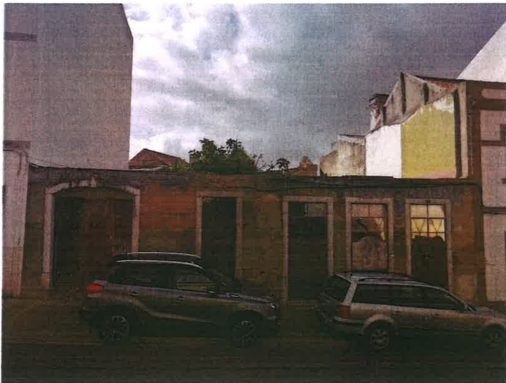
(foto 1) – Fachada principal
