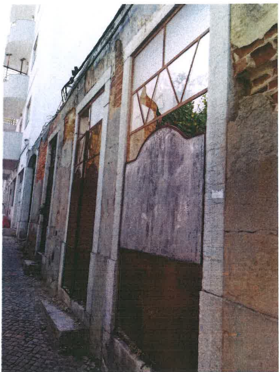
(foto 2) – Fachada Principal
